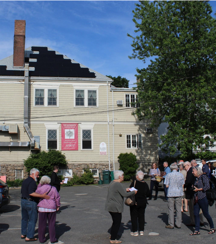
St. John's Episcopal Church, Gloucester, 11kW
