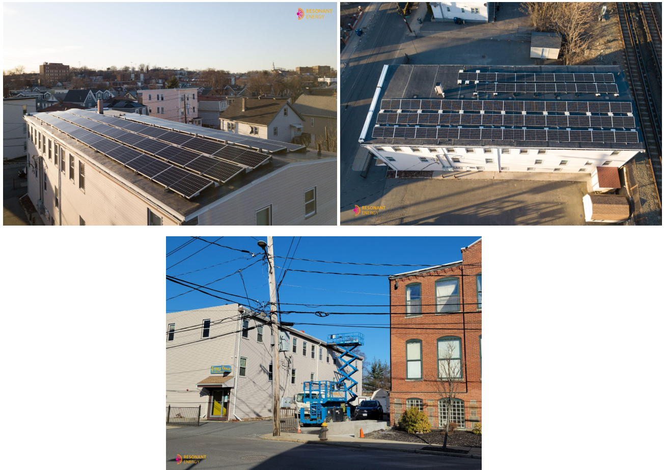
Top: The complete 23 kW DC solar array on the roof of MUA.
