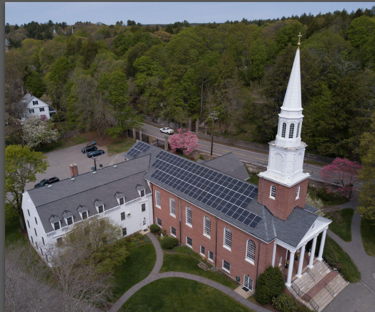
St. Peter’s Episcopal Church (CollectiveSun Solar Power Agreement 30 kW-DC)
