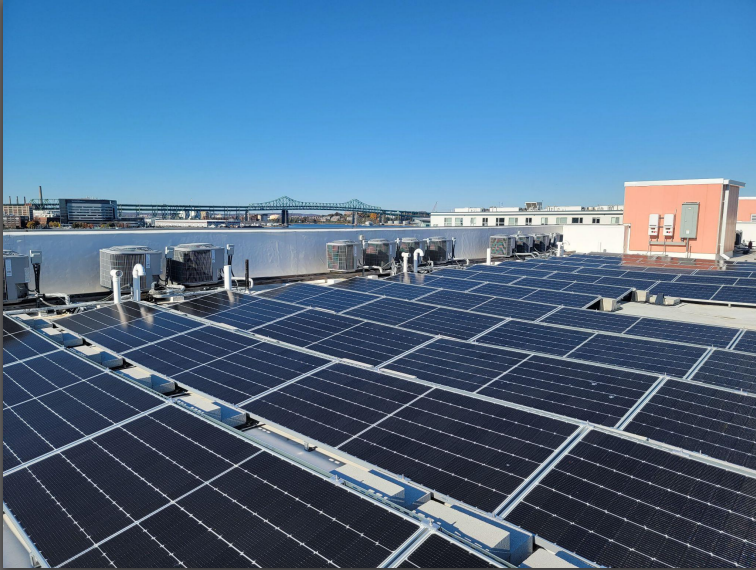
Coppersmith Village - Neighborhood of Affordable Housing
